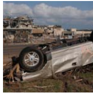
Ruins of Tornado-Ravaged Hospital to be Demolished
